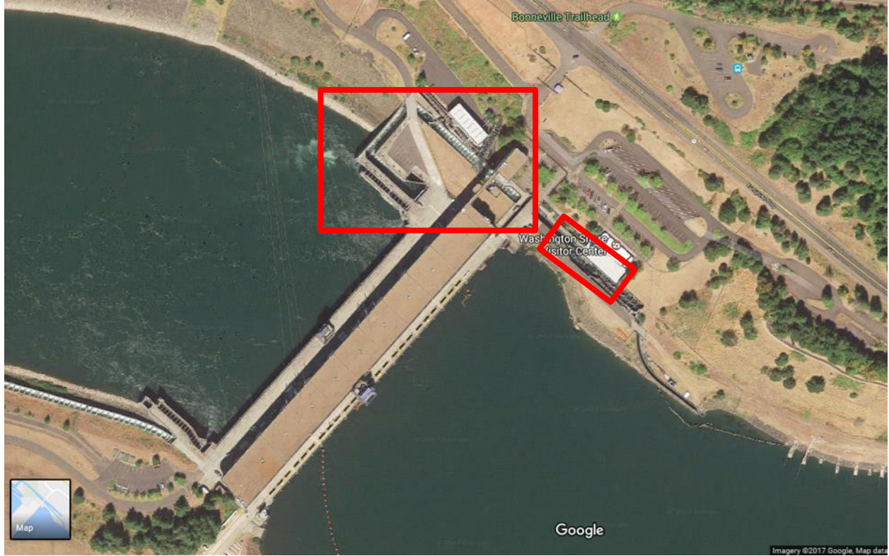
Figure 2. Close-up aerial view of Bonneville Dam with the Adult Fish Facility and upper Washington Shore Fish Ladder outlined in red boxes.
