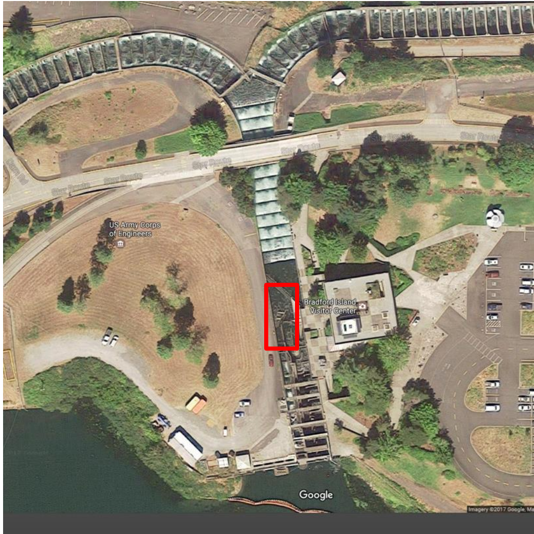
Figure 5. Close-up aerial view of the Bonneville Dam Bradford Island Fish Ladder at the count station and visitors center. Potential trap locations above picketed leads are outlined by red box. Alternate locations may be selected upon consultation between USACE and CRITFC member Tribes.
